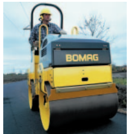
BW90AD-2 in action on an asphalt repair
