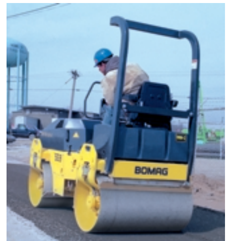
BW120AD-3 in action on chip and seal application.
