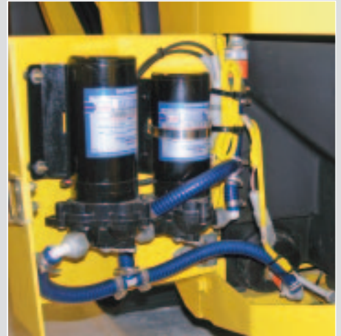
Dual water spray pumps, providing back-up provision.
