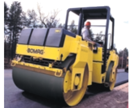
BW151AD-2 in action on highway construction
